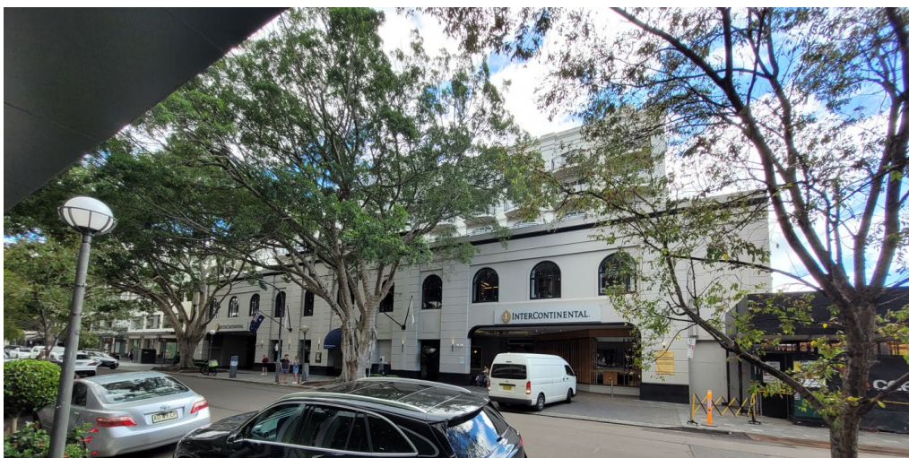
View of the subject site from Cross Street
