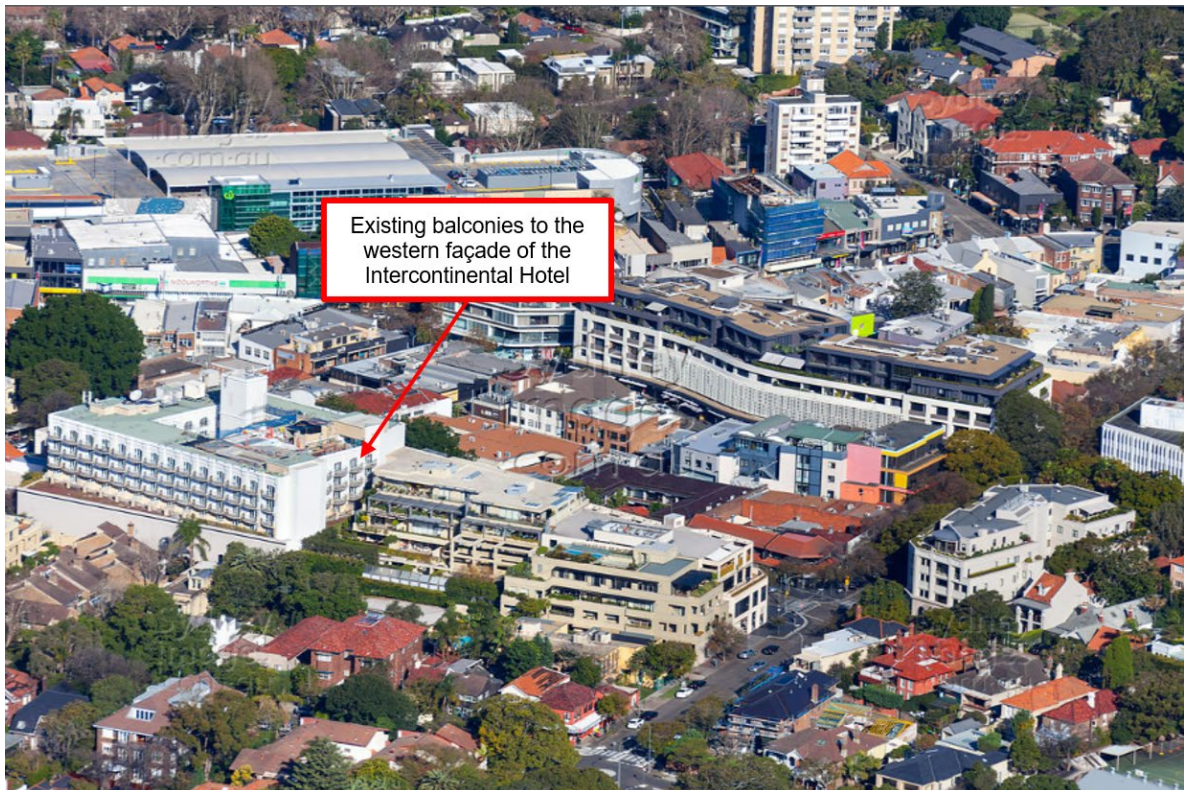
Aerial view showing the existing balconies to the western façade of the Intercontinental Hotel (Source: Double Bay Aerial Photography)
