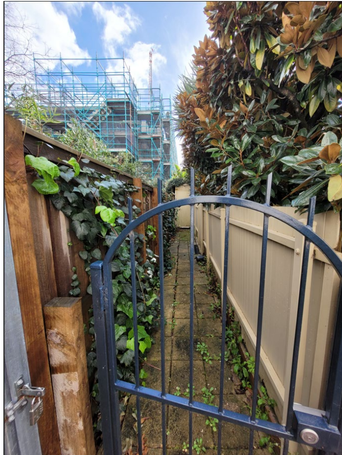
View looking in a northerly direction towards the rear of No. 27-29 William Street (RFB currently under construction). The development on the right-hand side of the private access lane is 31-33 William Street
