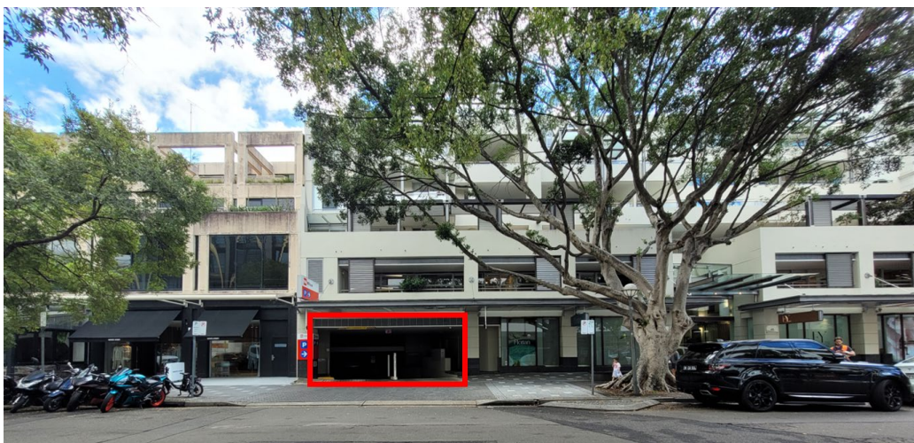
View of the existing access to the basement parking of the subject site located at Nos. 45-51 Cross Street
