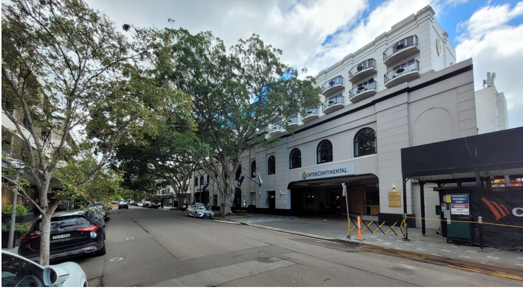
View of the subject site from Cross Street
