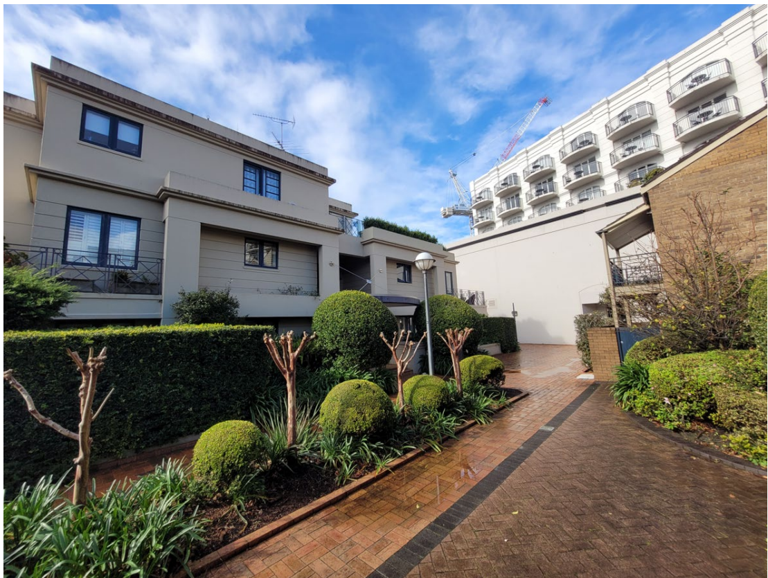
View of the subject site from Galbraith Walkway with the southern part of the development at No. 35-39 William Street located in the foreground, showing the separation between the subject site and adjoining development to the north
