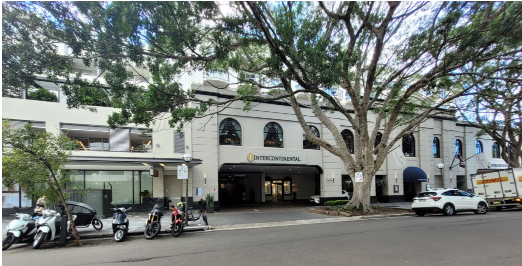
View of the subject site from Cross Street
